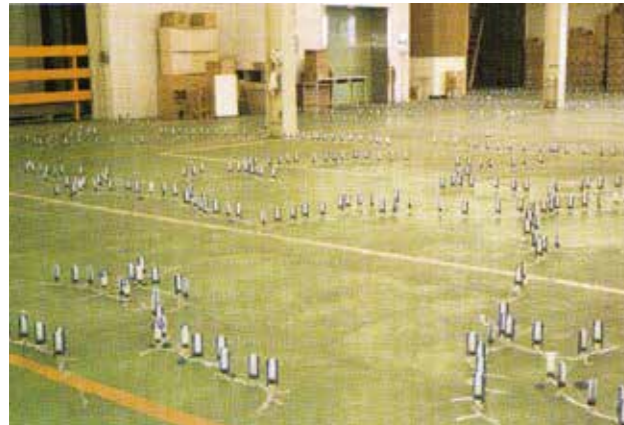
床ひび割れ補修
